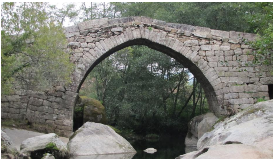
Fig. 3. 33 - Downstream side photo
