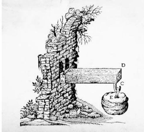
Fig. 2. 5 - Galileo's failure analysis (Benvenuto, 1981)
