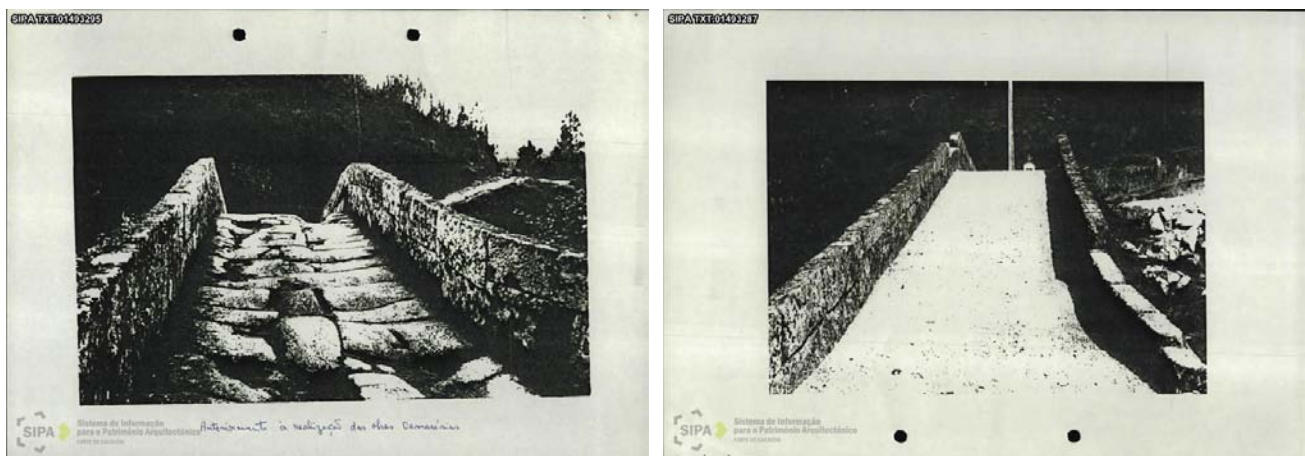
Fig. 3. 6 - Pavement intervention: a) before; b) after (SIPA)
