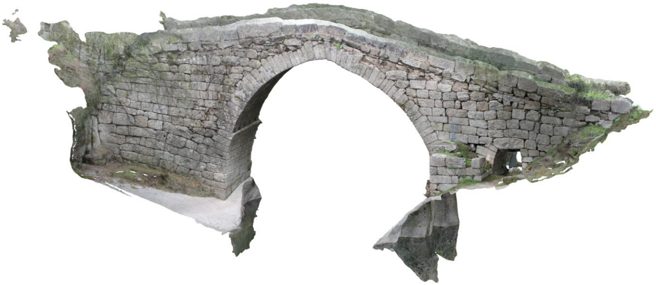
Fig. 3. 25 - 3D final model by PhotoScan
