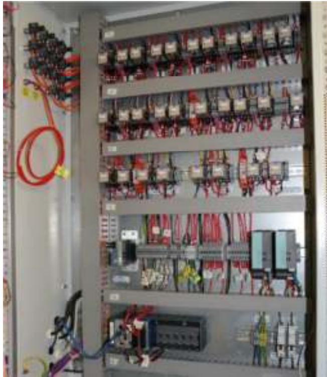
Fig 2.23: The control box connections
