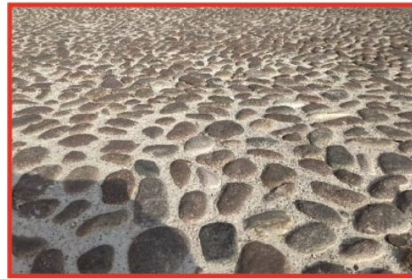
Figure 4.101 :Cobblestone surface tested, Via del Portello, Padova
