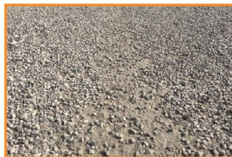
Figure 4.99: Gravel surface tested, Lungargine del Piovego, Padova
