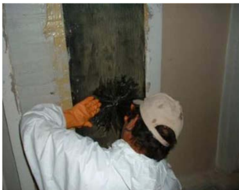
Figure A1.10 - phases of FRP installation
