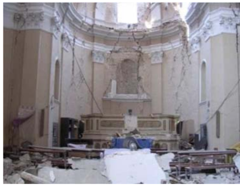
Figure A1.11 - apse collapse
