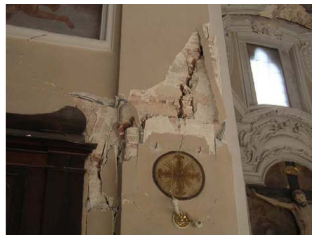
Figure A1.18 – Out-of-plane movement of the chapel walls.
