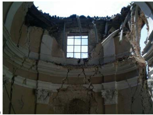
Figure A1.11 - apse collapse
