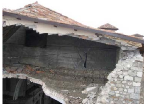
Figure A1.14 - RC tympanum collapse
