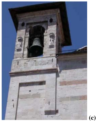
Figure A1.6 - new bell towers roof
