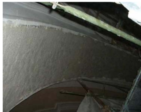
Figure A1.10 - phases of FRP installation
