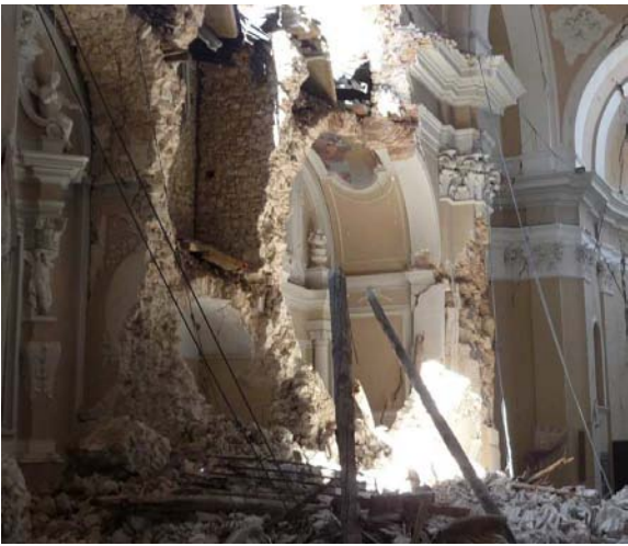
Figure A1.21 – Chapels vaults collapse.
