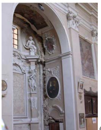
Figure A1.18 – Out-of-plane movement of the chapel walls.
