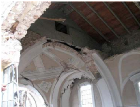
Figure A1.14 - RC tympanum collapse
