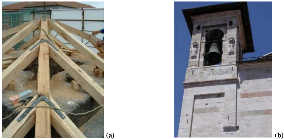
Figure 3.13 - New bell towers roof.
