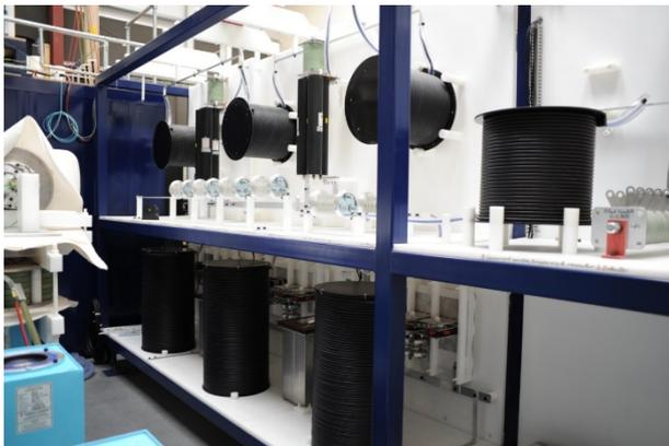
Figure 4.14 - Transit filter in the B/C-bank
