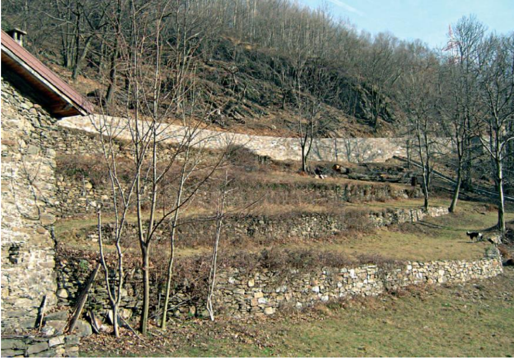
Figure 2.7. Terraces in Adamello Park (picture from Sangiorgi et al., 2006).
