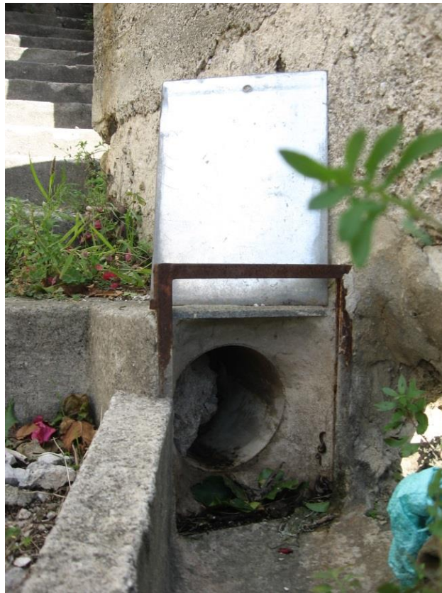
Figure 3.25. Disused bulkhead in a channel in Minori.
