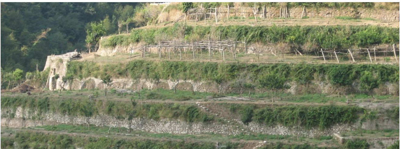
Figure 3.20. Terraces with supporting arches in Maiori. The area was abandoned but now is under restoration.
