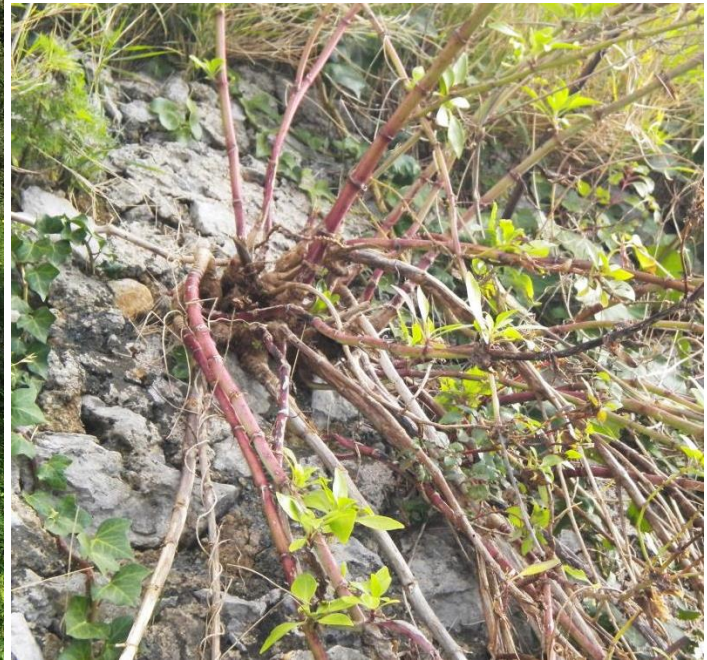
Figure 4.9. a) bulging in the wall middle part in Cetara; b) wall top degradation due to arboreal invasive vegetation growth.
