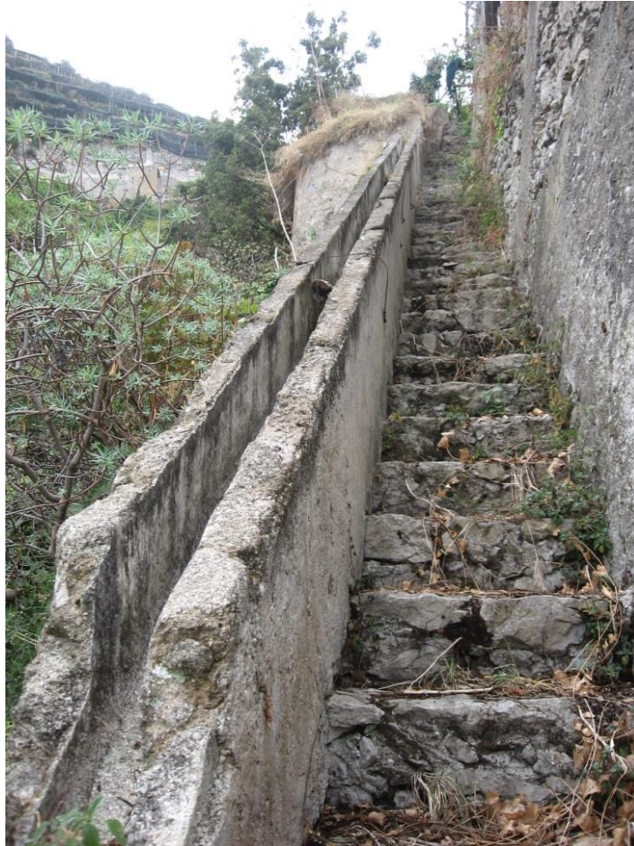
Figure 3.26. Water conduit on a handrail at the side of a stairway in Maiori.
