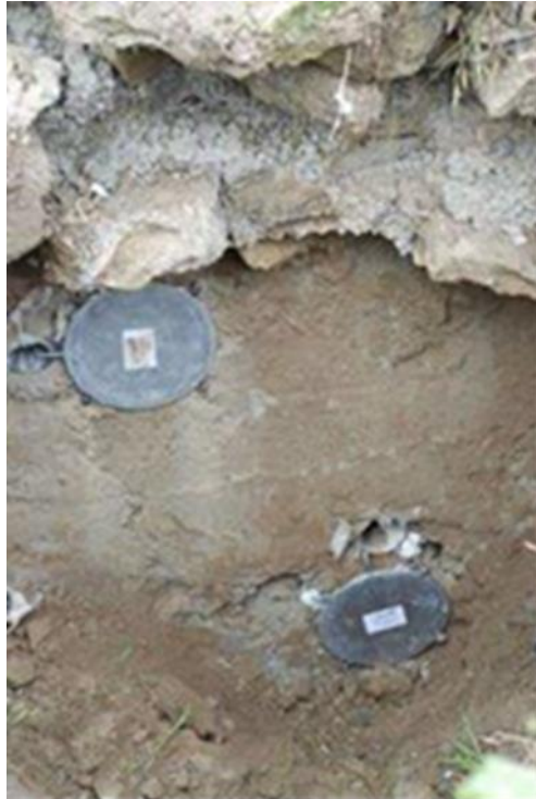
Figure 5.30. Total pressure cells installed behind the wall in Lamole, Chianti.
