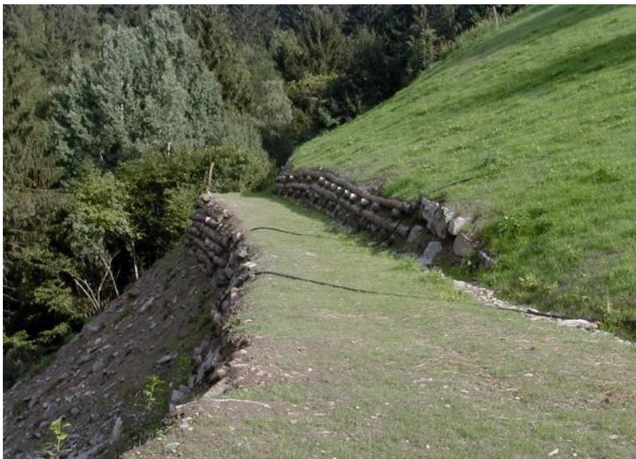
Figure 5.21. Slope restored with a wooden cribwall (original picture from D'Agostino, 2013).
