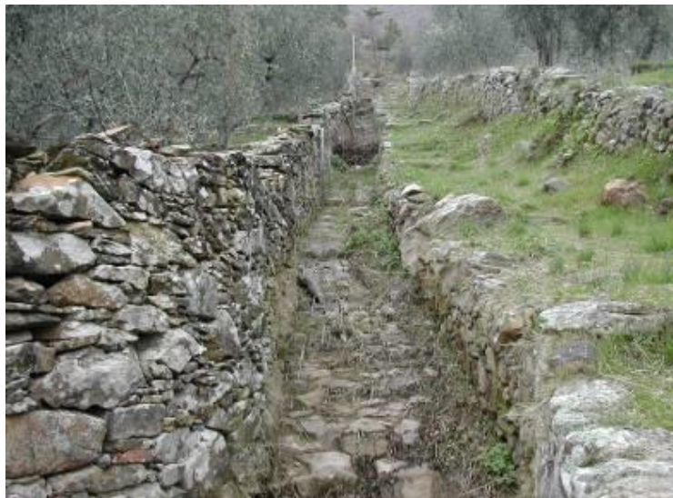
Figure 5.10. Channel for surface water drainage in Tuscany (picture from Rizzo et al., 2009).
