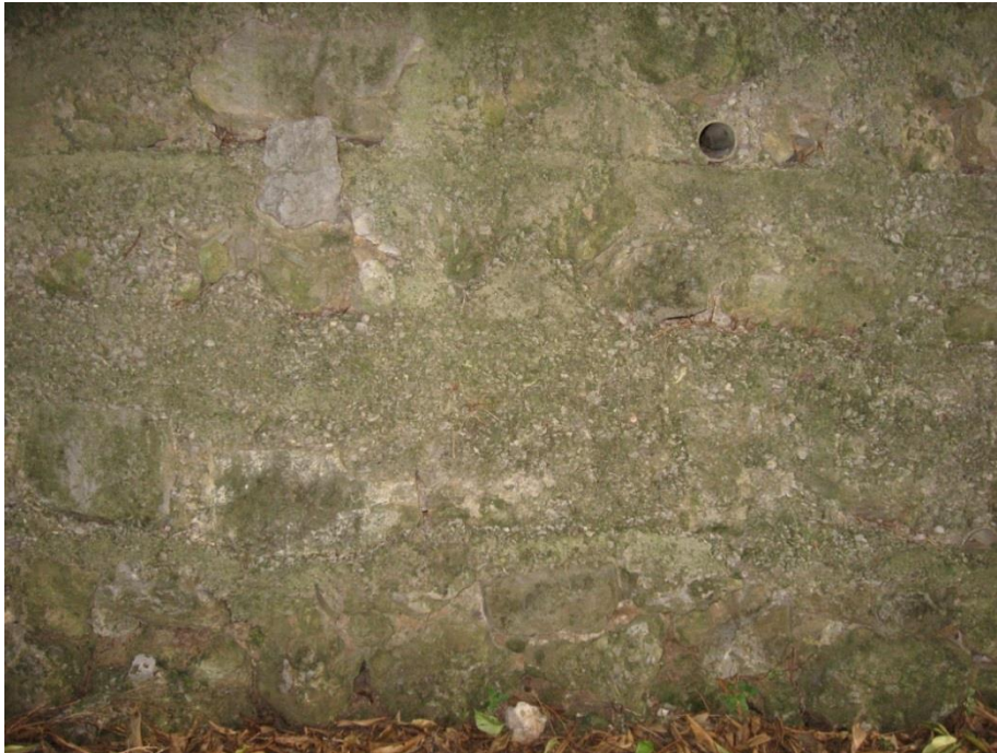
Figure 3.23. Terrace wall repaired with concrete in Tramonti.
