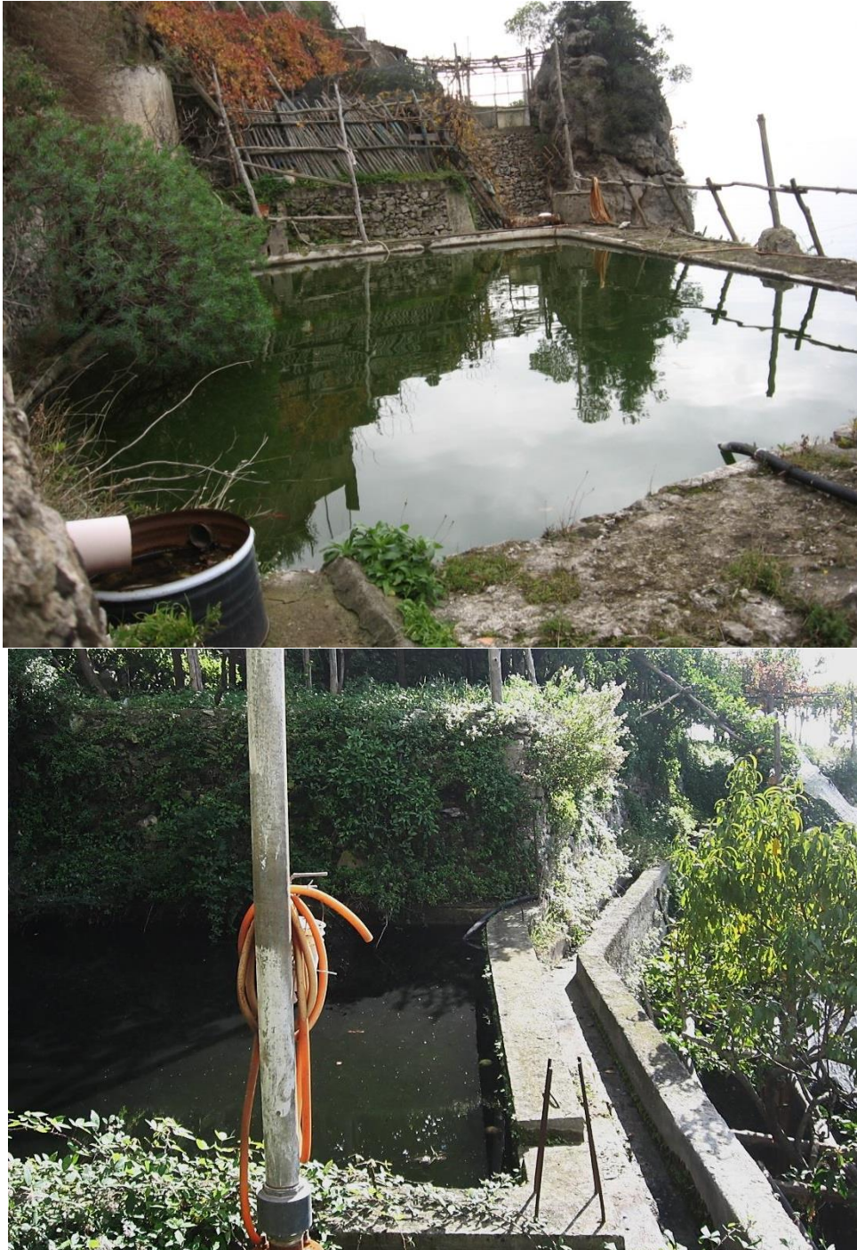
Figure 3.27. a) pool for water collection for irrigation in Maiori; b) water pool and Minori, it can be noted the mortar channel for redistribution of water in excess on the terraces.
