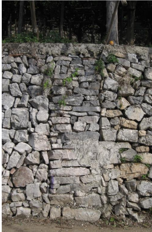
Figure 3.17. Flat stones in shape of piers in the middle of terrace walls in Minori.
