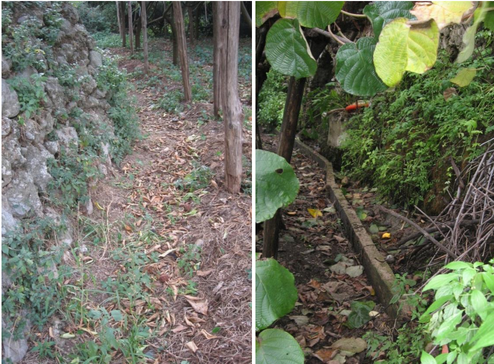
Figure 3.28. a) lavinari at the bottom of a terrace in Tramonti; b) lavinari with wooden supports at the bottom of a terrace in Maiori.
