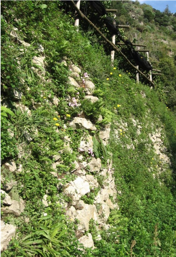
Figure 4.9. a) bulging in the wall middle part in Cetara; b) wall top degradation due to arboreal invasive vegetation growth.
