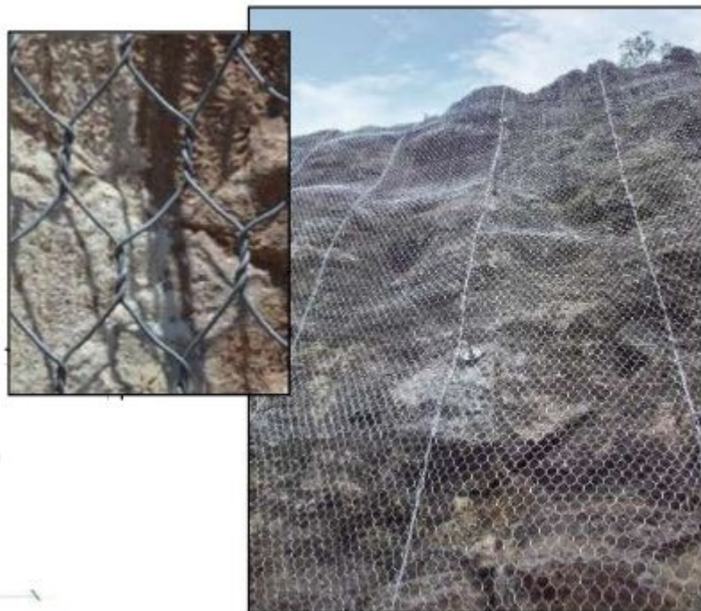
Fig 1.5: Double twisted wire mesh
