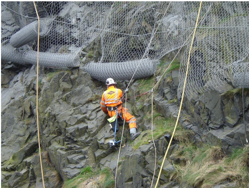
Fig 1.14: Secured drapery system installation
