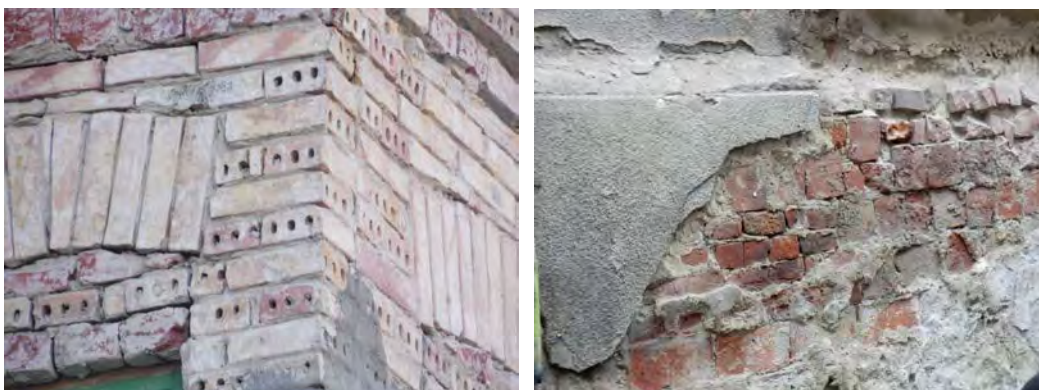
Fig. 1.9.3: Holed bricks and irregular masonry (US 5 and US167)
