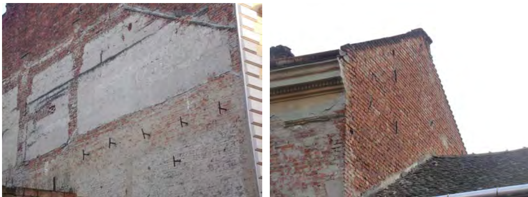
Fig. 1.10.3: Tie rods examples(US 79 and US 237)
