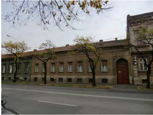
Fig. 1.8.11: Passage to the internal courtyard (US 210)
