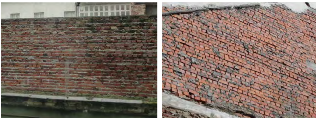
Fig. 1.9.2: Uprising masonry (US 100 and US 85)
