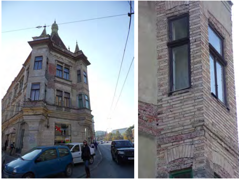
Fig. 1.8.4: Overhanging elements and holed bricks(US 5)
