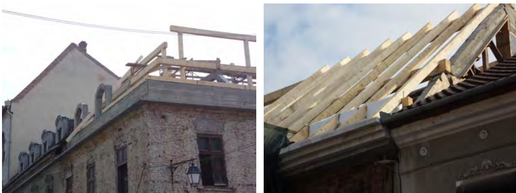
Fig. 1.9.20: Non –thrusting mixed roof examples (US 82)
