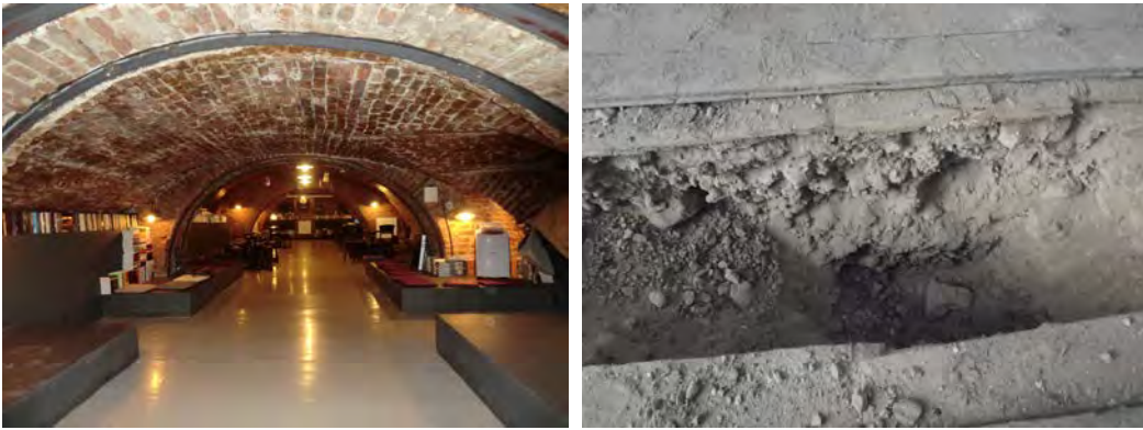
Fig. 1.9.12: Brick vault example and soil and shard filling (US 192 and US 130)
