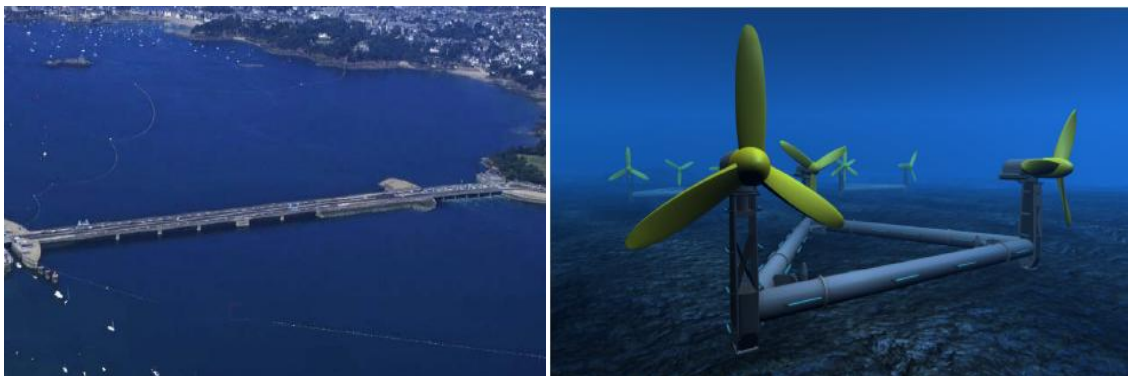
Figure 1.1 a) "La Rance" tidal turbine power plant [2] (left), b) DeltaStream tidal turbine [4] (right)
