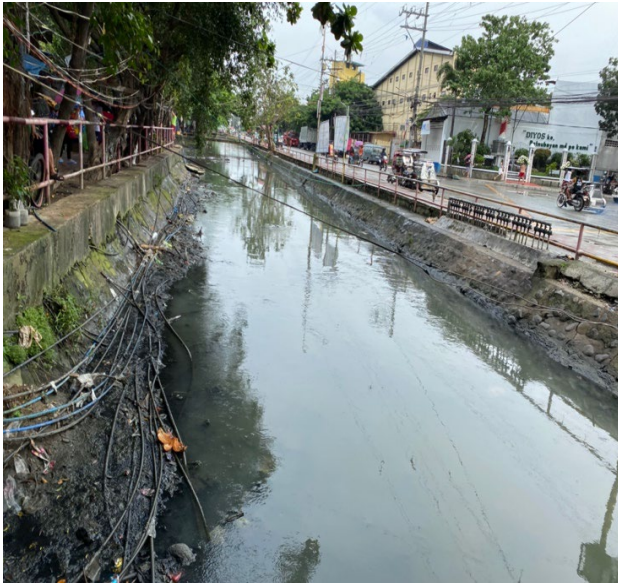
Figure 6. Laying down pipelines on public land.
