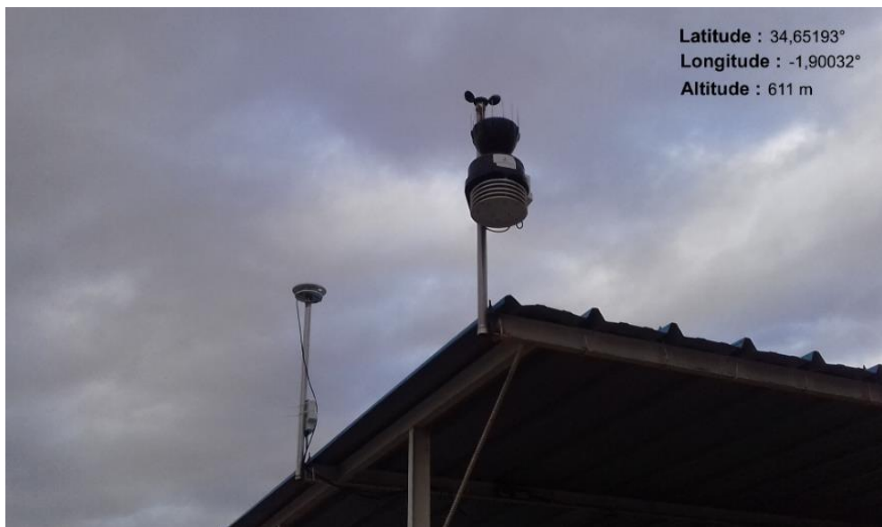
Figure 3. Installation site of the weather station.
