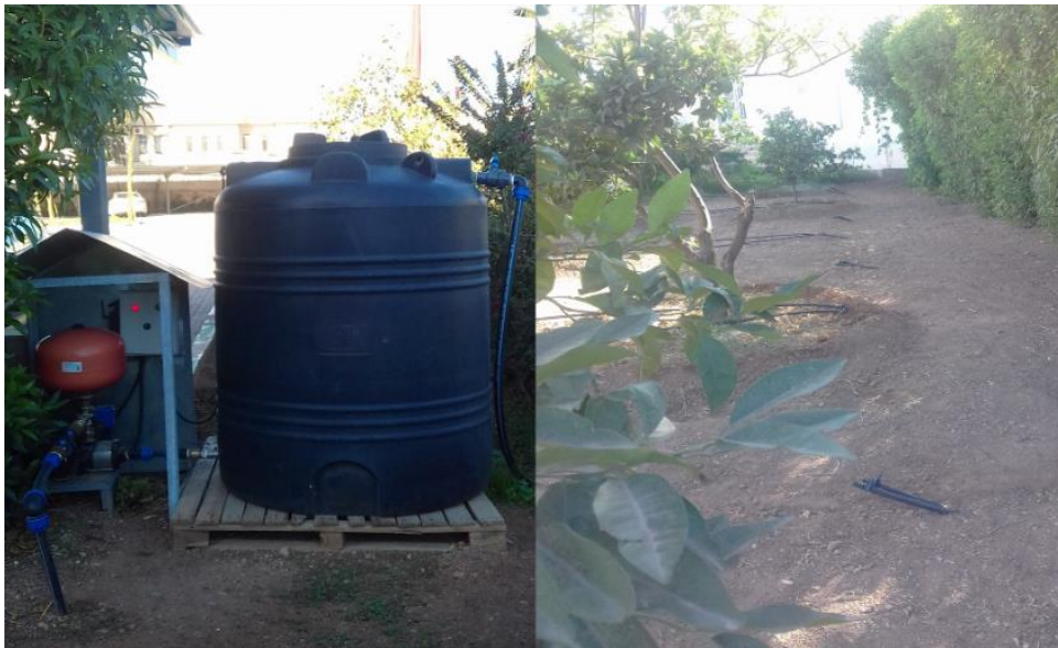
Figure 2. Installation of irrigation equipment.
