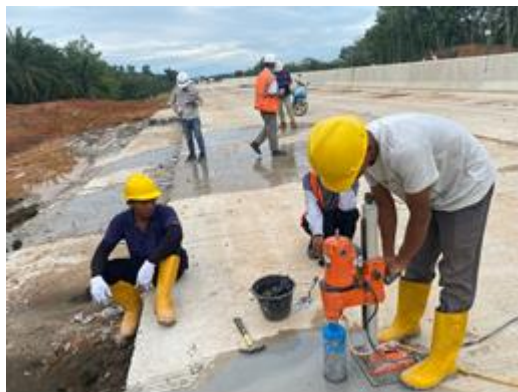
Gambar 3.27 Pengujian Core Drill
