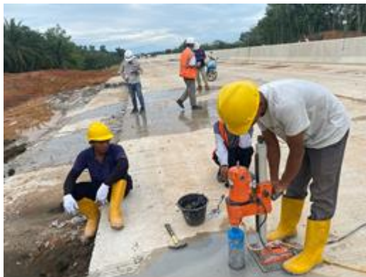
Gambar 3.10 Pengujian Core Drill
