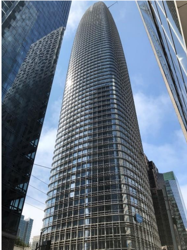
Figure 5.2 Glass Curtain Wall Nearing Completion.
