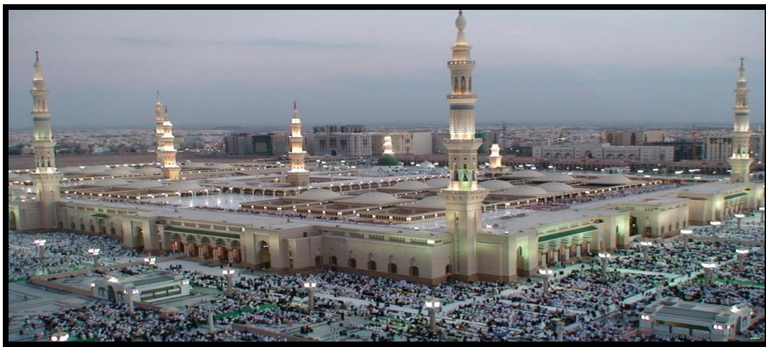
Figure 6. Corner view of the Prophet Mosque (AGPPM).
