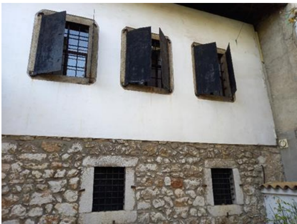
Figure 15. Ancillary room with massive stone walls (Source: authors)
