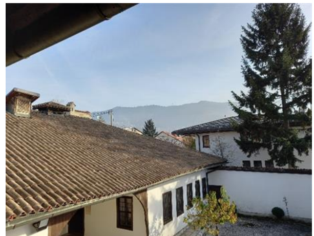
Figure 16. Sloped roof with hollow tiles covering (Source: authors)
