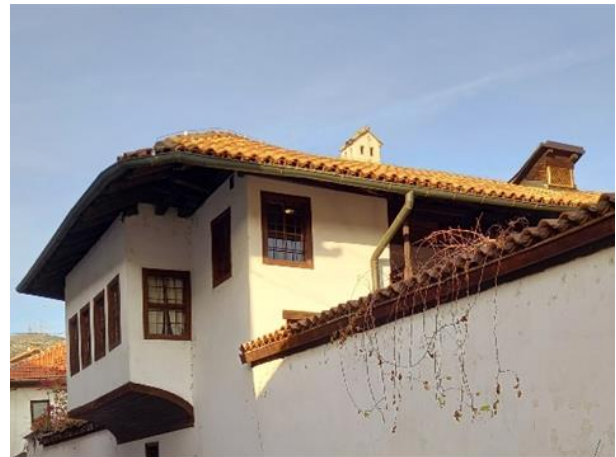
Figure 14. Doksat overhanging the street (Source: authors)
