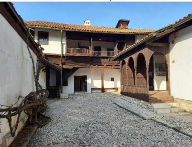
Figure 9. Selamluk with courtyard (Source: authors)
