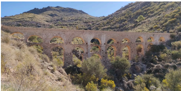
Figure 2. Current state of conservation of the aqueduct
