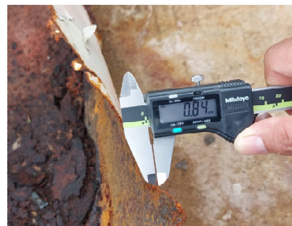
Gambar 6. Pengukuran ketebalan dinding ducting
