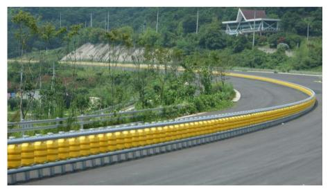
Fig. 4 - Roadside rolling barrier at hilly road [15]
