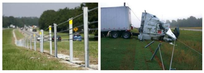
Fig. 8 - Cable barrier [12]
