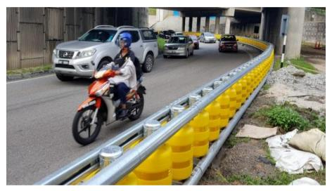
Fig. 3 - Roadside rolling barrier at curved road [14]
