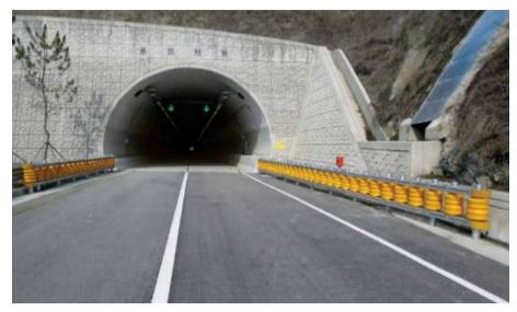
Fig. 2 - Roadside rolling barriers at straight road [13]
