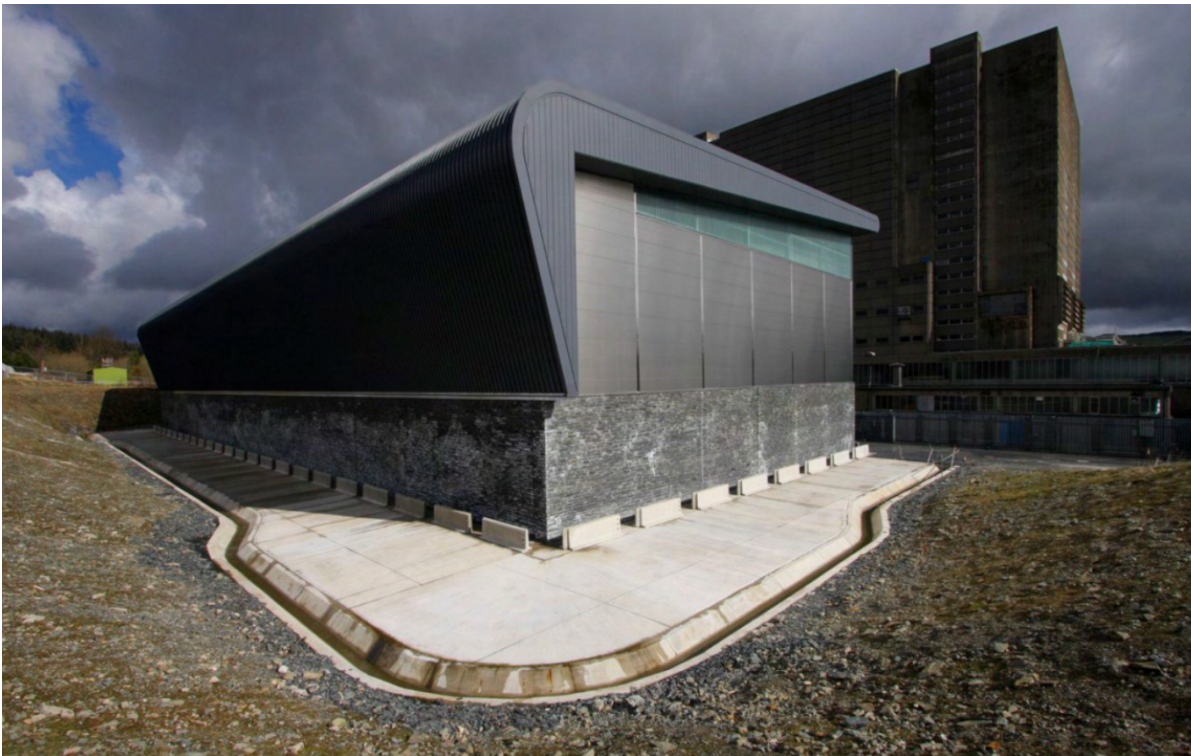
Figure 1.3: Photograph of the Trawsfynydd ILW Store, taken from [62]. Locally mined slate was used on the exterior of the building to improve the aesthetics and support the local economy.
