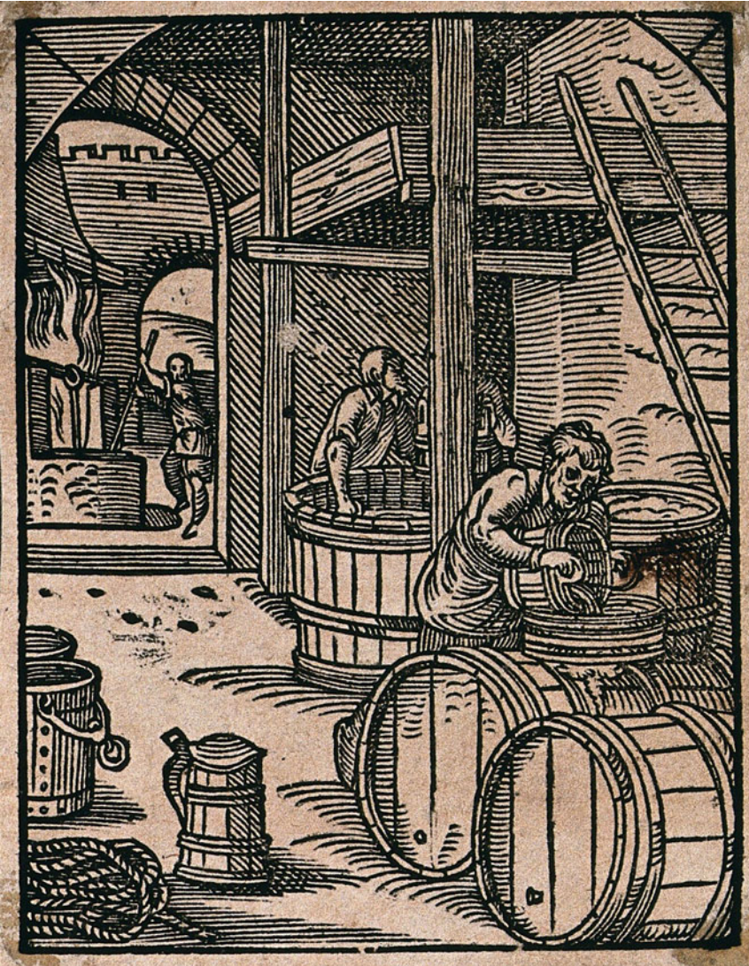
Figure 4. A sixteenth-century brewhouse.
