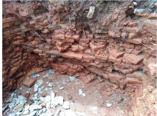
Figure 7. Level 2, corner of brick plinth covered with stucco (left). Layers of brick (right). Photographs by U Min Aung ( CC BY-NC 4.0 ).
