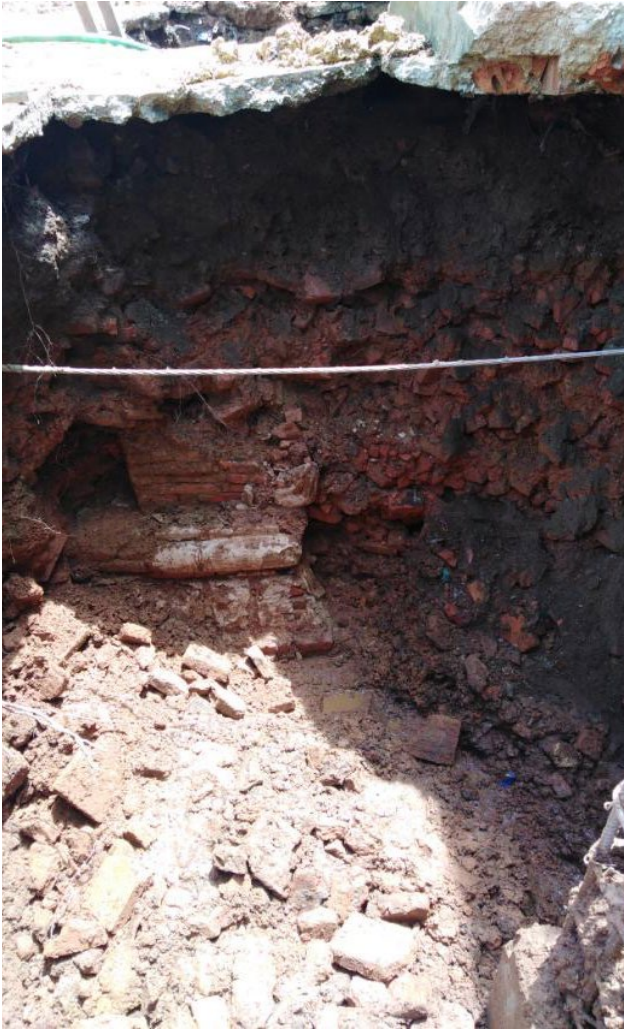
Figure 7. Level 2, corner of brick plinth covered with stucco (left). Layers of brick (right). Photographs by U Min Aung ( CC BY-NC 4.0 ).
