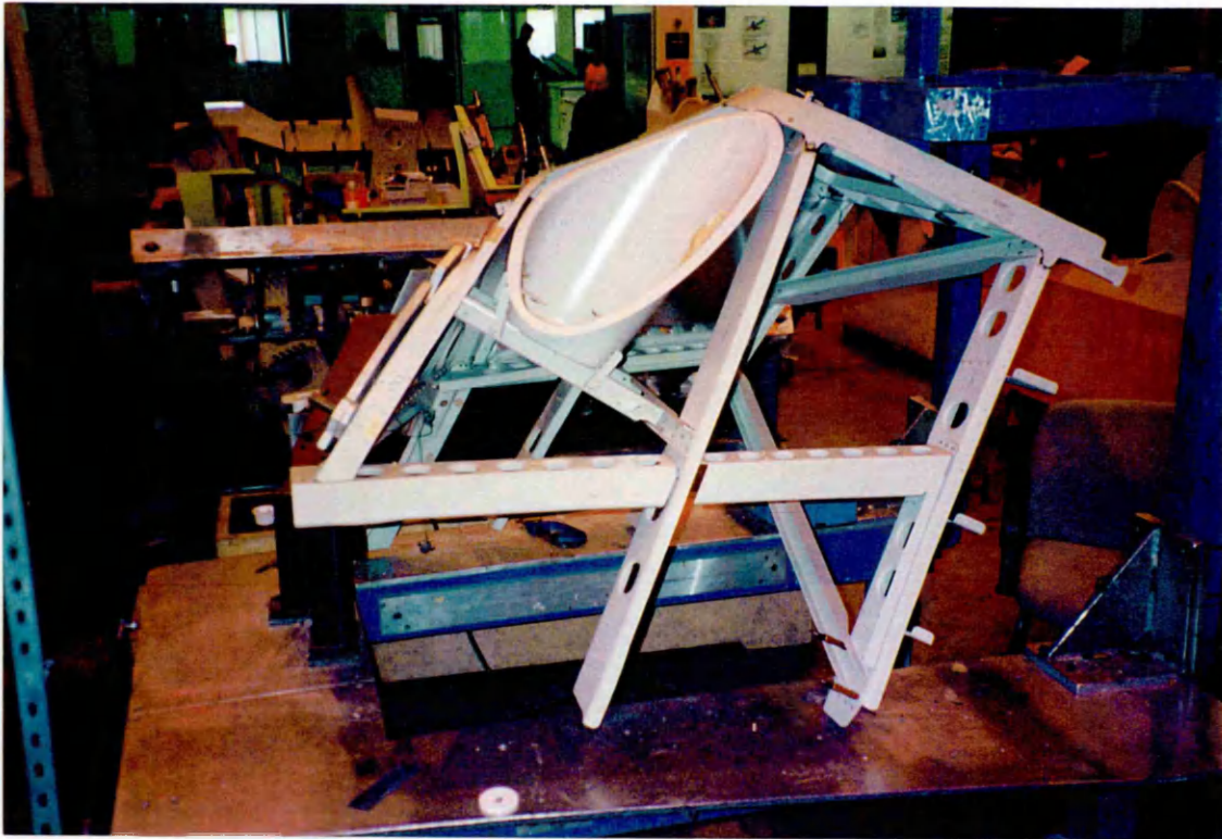
Figure 6.2.2.5. Frame work re-assembly in stage 02 assembly fixture
