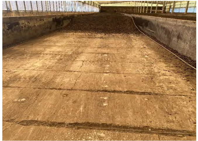
Figure 6. Air supply pipelines are installed at the bottom along the compost pit row and are not operating because the mixing vessel created enough aeration, and the aeration requires a lot of maintenance.
