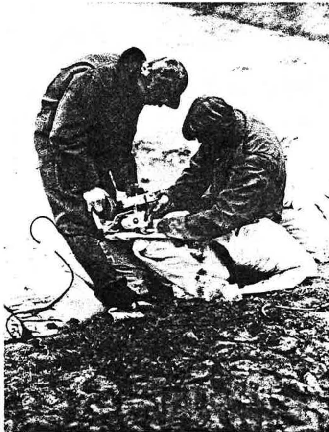
Figure 22. Finishing the Seam .
