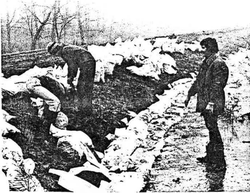
Figure 23. Positioning the Bags on the Dam
