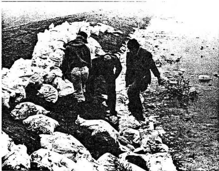
Figure 24. Positioning the Slope Protection System
