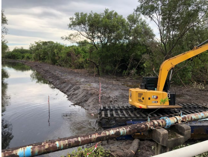
Fig. 3.5: Dredging carried out by Department of Irrigation and Drainage (DID), Sarawak at Sungai Lutong to deepen the channel.
