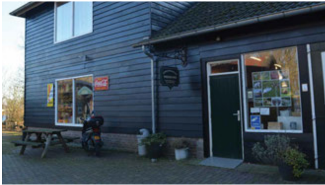
Entrance | needs improvement
