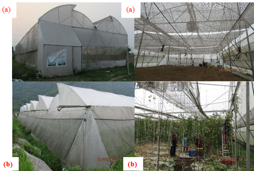
Figure 3. Semi Hi-tech poly-house (a) Naturally ventilated double span (b) Naturally ventilated multi-span
