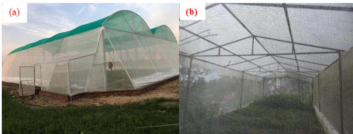
Figure 5. (a) Net House (b) Screen house with its all features installed in farmers field
