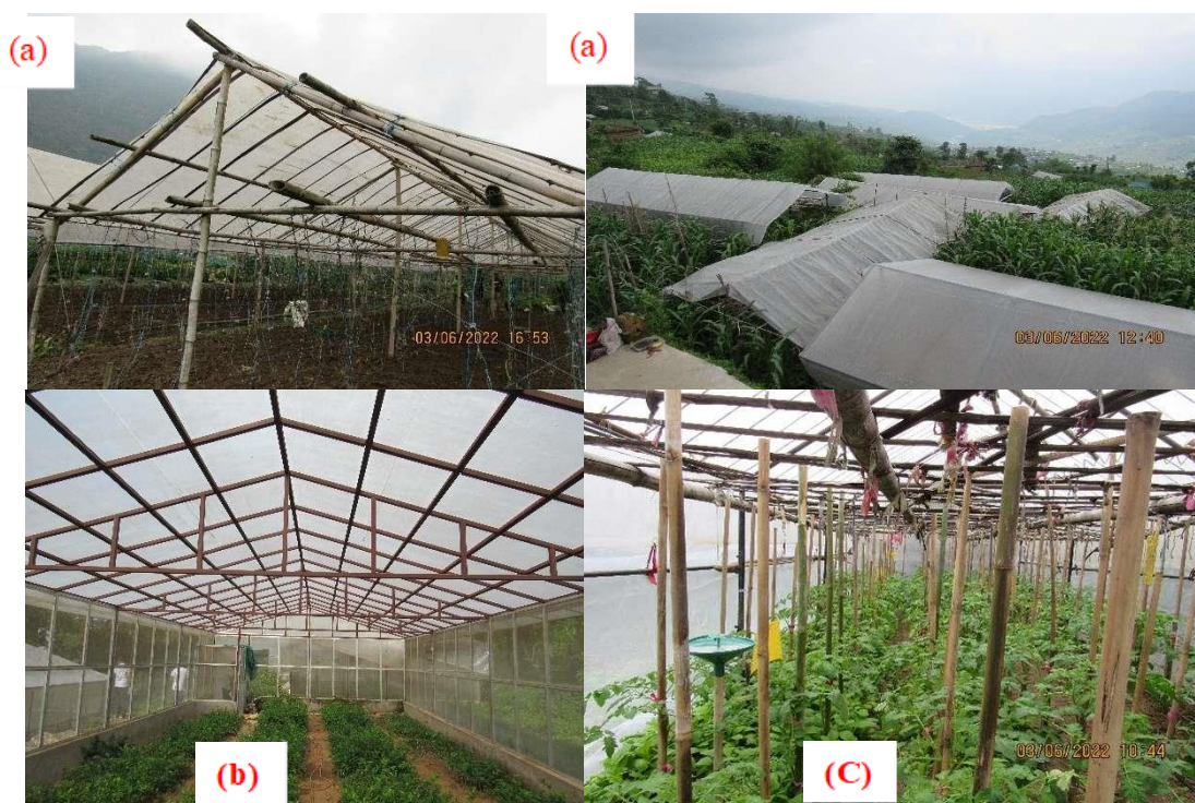
Figure 2. Low cost plastic (a) Bamboo open shed (b) GI framed tunnel (c) Bamboo tunnel
