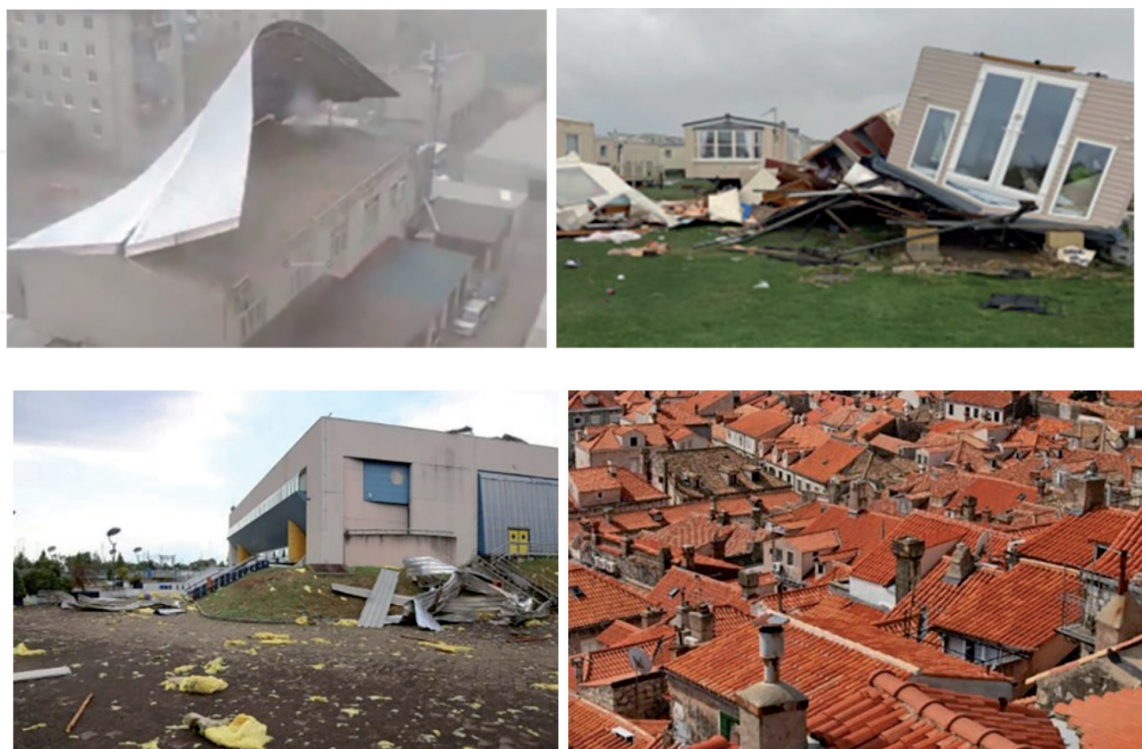
Figure 3. The environment assessment is essential to identify the possible risks and the elements that can fail in case of strong winds, becoming flying debris.
