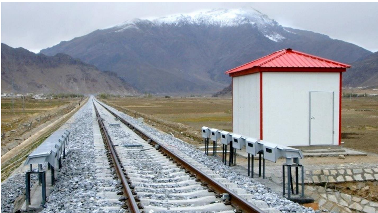
Figure 4: Photograph of Trackside Acoustic Detection System site [10]
