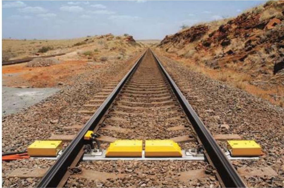
Figure 5. On-site Hot-Box-Detector (HBD) system [5]
