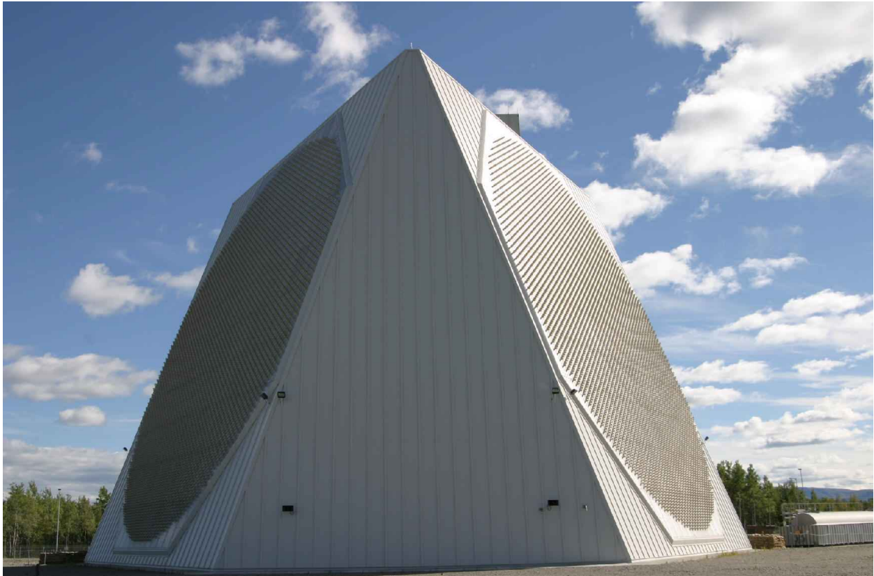
Figure 1.3: The Precision Acquisition Vehicle Entry Phased Array Warning System (PAVE PAWS) at Clear Air Force Base in Alaska was built for the U.S. Air Force in the 1970s with a total of 2,677 crossed-dipole elements in two circular arrays.
