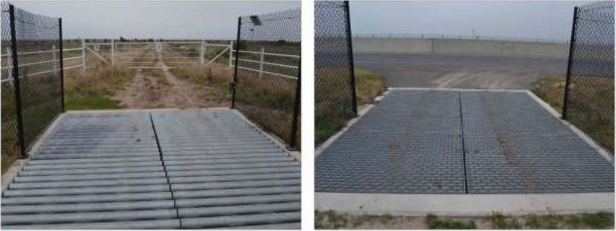
Figure 3. The two wildlife guard (WG) types constructed by the Texas Department of Transportation to address ocelot ( Leopardus pardalis albescens ) mortality along State Highway 100 in Cameron County, Texas, USA: pipe (left) and bridge grating (right). WG were monitored using remote cameras, and data were collected at these sites from April 2017 to May 2019.
