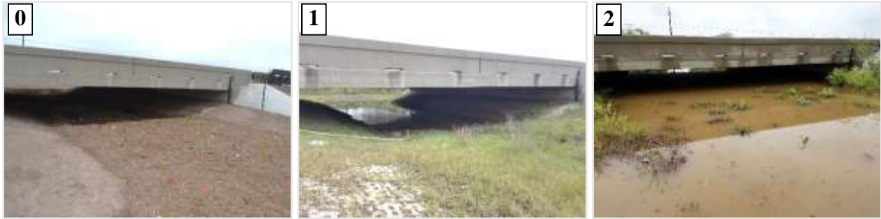
Figure 14. Water inundation at one wildlife crossing structure, located on State Highway 100 in Cameron County, Texas, USA, occurring between January 2018 and May 2019: little to no water (0); intermediate pooling of water (1); full of water (2).
