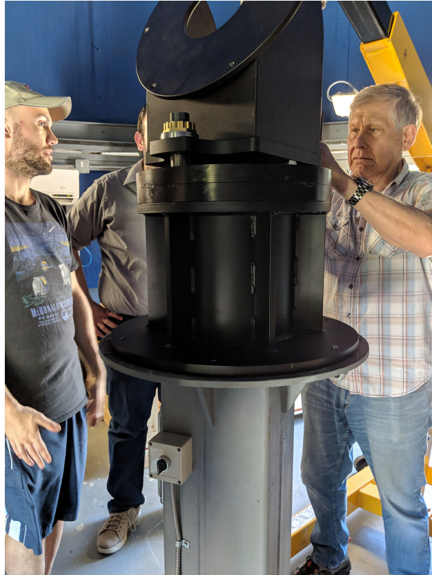
Figure 3.6: Pedestal, pier, and wedge before installation of mount
