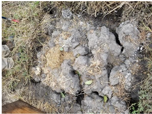
Figure 18. Cover board with extreme soil desiccation underneath.
