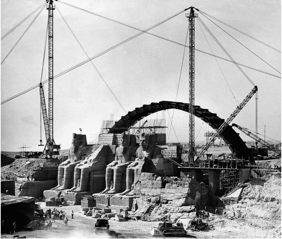
Figure 8, View of the Structures Required to Lift the Monuments out of the Path of Flooding Caused by the Aswan High Dam, Terrence Spencer
