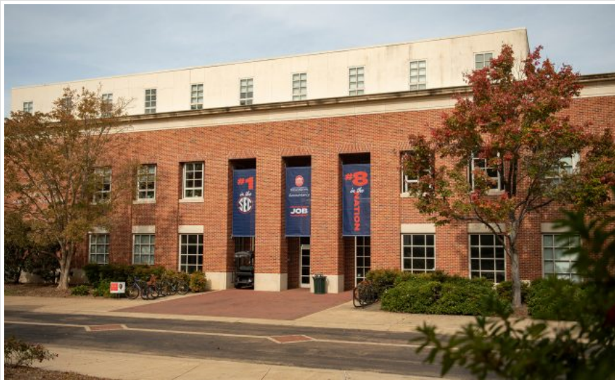
Thanks to private gifts from donors such as Larry Hardy, the Patterson School of Accountancy will move from its longtime location in Conner Hall on Business Row to new construction at the corner of Grove Loop and University Avenue. Photo by Logan Kirkland/Ole Miss Digital Imaging Services
