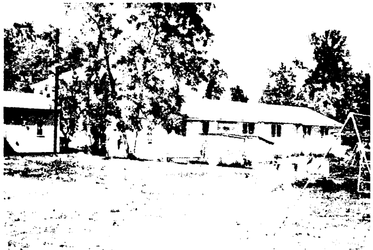
Rear view of school plant.
