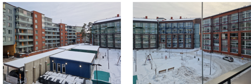
Figure 2.3.2.18 The outdoor condition on 28 th of Feb .
