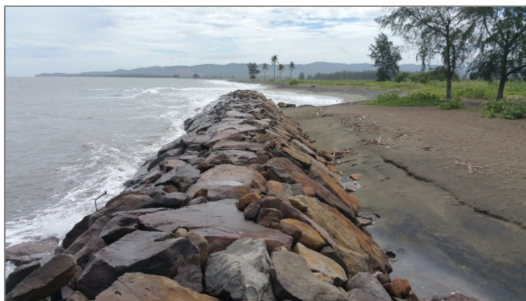
Figure 4. Condition of revetment point 6
