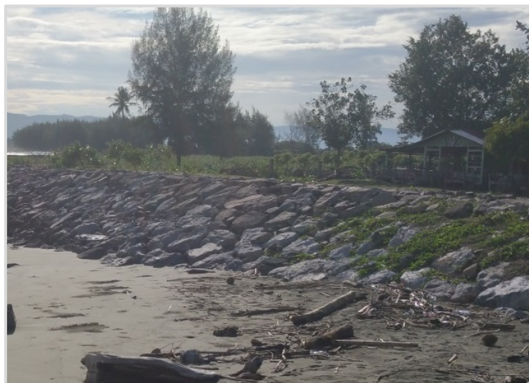
Figure 3. Condition of revetment point 1
