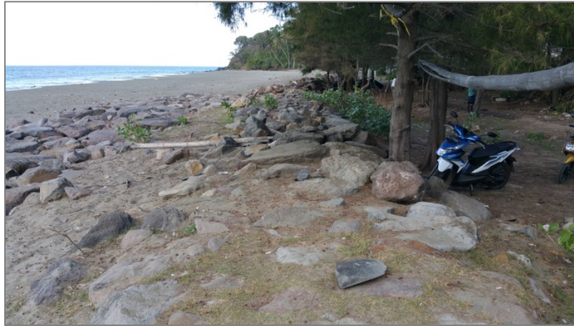
Figure 10. Condition of building jetty at point 8
