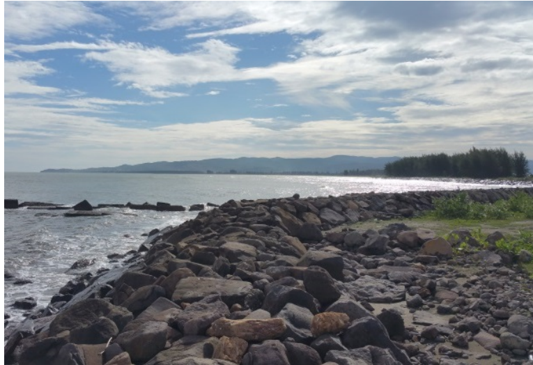
Figure 5. Condition of revetment on the track 2
