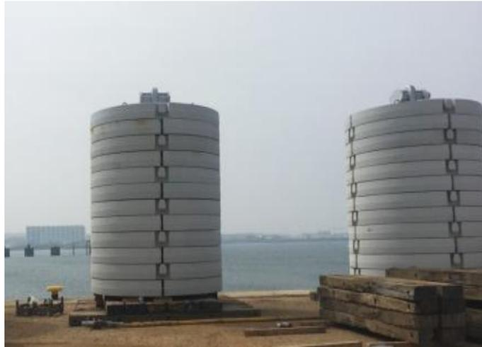
**Figure 2.12:** Gravity anchors (Group, n.d.)
