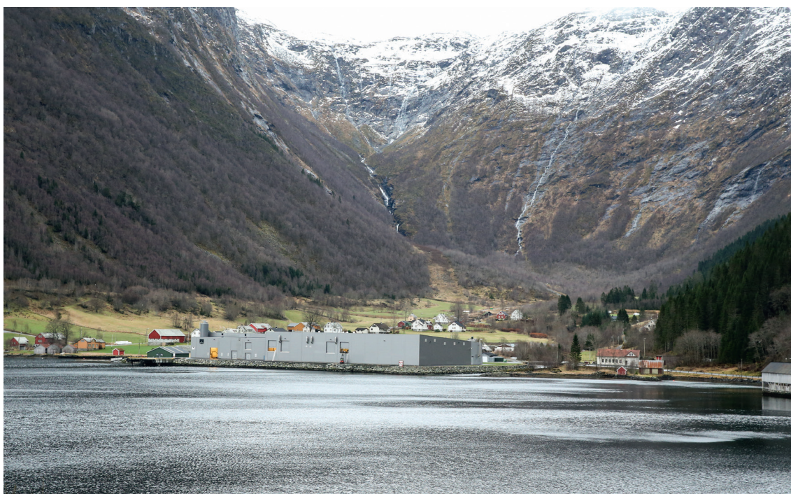
MOWI's RAS tech smolt plant facility in Steinsvik, Norway. Photo: © MOWI
