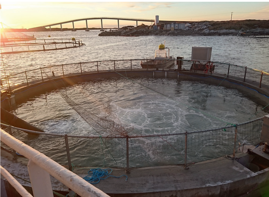
Pilot cage of 1.000 m 3 floating semi-closed concrete sea cage at Gullklakken. Photo © Nekton
