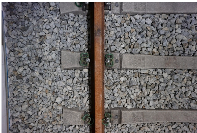
Fig. 4. Image of the railway track.
