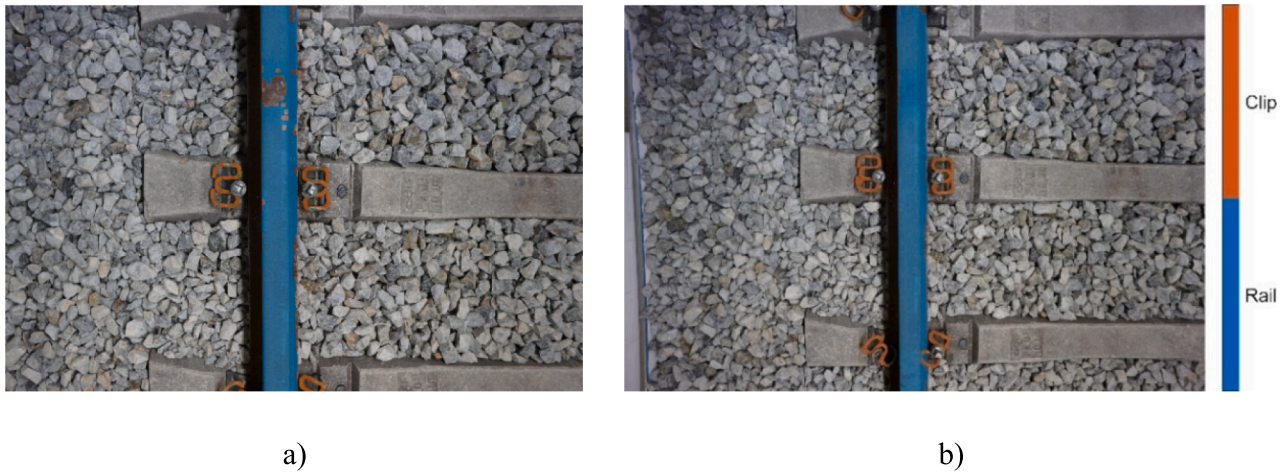
Fig. 6. Clip and rail segmentation. a) Colour segmentation. b) Morphologically closed segmentation.
