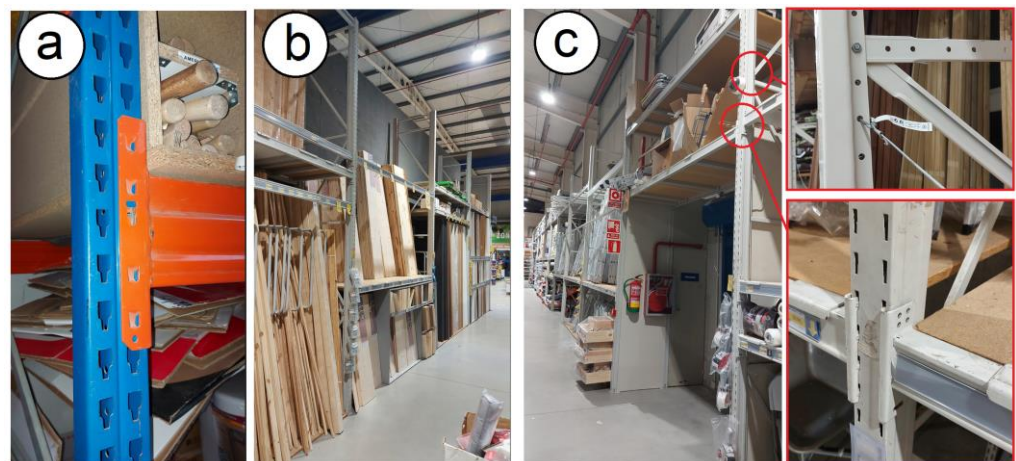
Figure 5. (a) Beam–end connection to perforated profile column in steel storage racks, (b) load-bearing structure made of steel racking, and (c) steel racking from perforated profiles.
