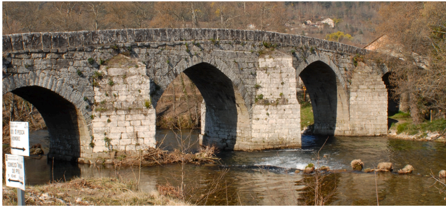
Fig. 1. Overall view of Cernadela Bridge.
