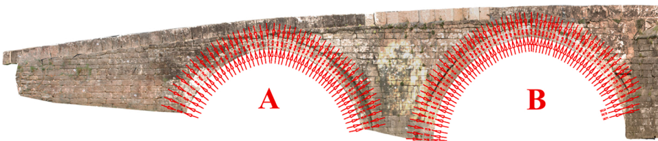
Fig. 6. Experimental measurement of the arches' outer thicknesses.
