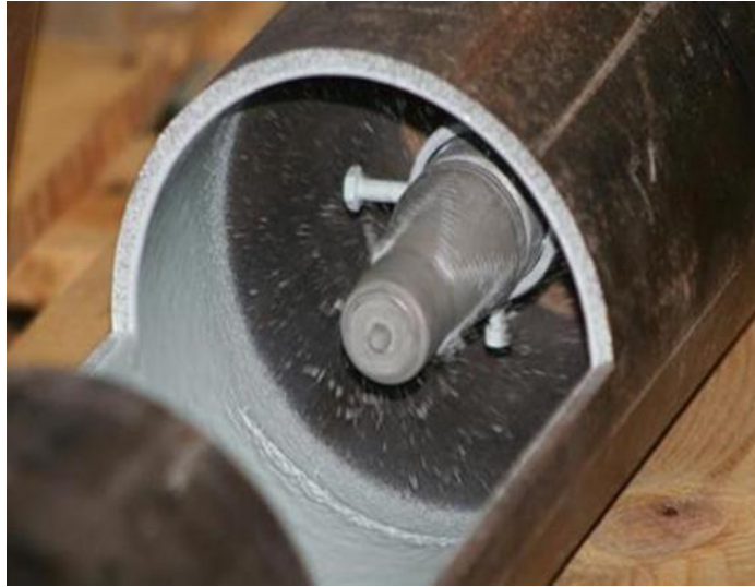
Figure 2-15: Epoxy pipe lining – Courtesy Trenchless Pipe Lining
