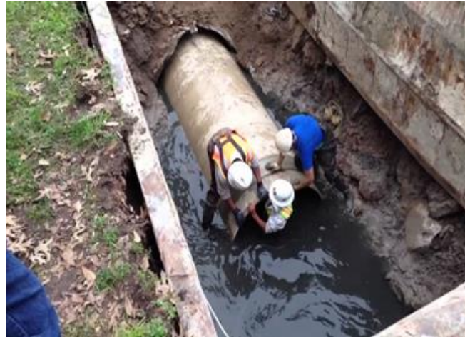
Figure 2-8: Sliplining with flow – Courtesy mclewis888
