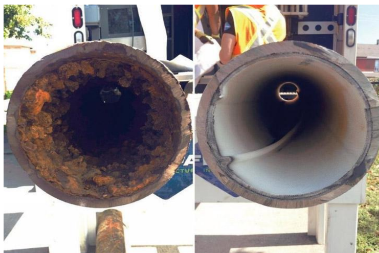
Figure 2-6: Water line repaired using CIPP - Courtesy Aquazen Services
