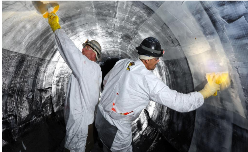
Figure 2-4: Manual application of FRP Liner - Courtesy Water News Network
