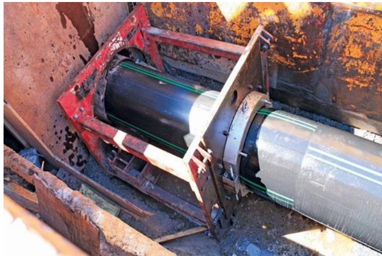
Figure 2-10: Installation of HDPE liner – Courtesy Trenchless Technology Magazine
