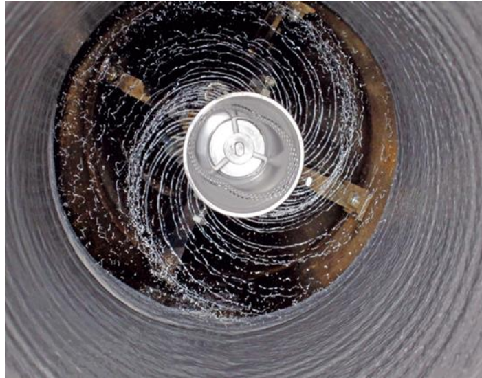
Figure 2-16: Centrifugal spray applying polyurea – Courtesy Trenchless Technology Magazine
