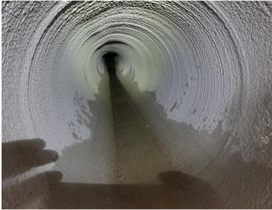
Figure 2-14: Geospray geopolymer liner post installation – Courtesy ClockSpring NRI
