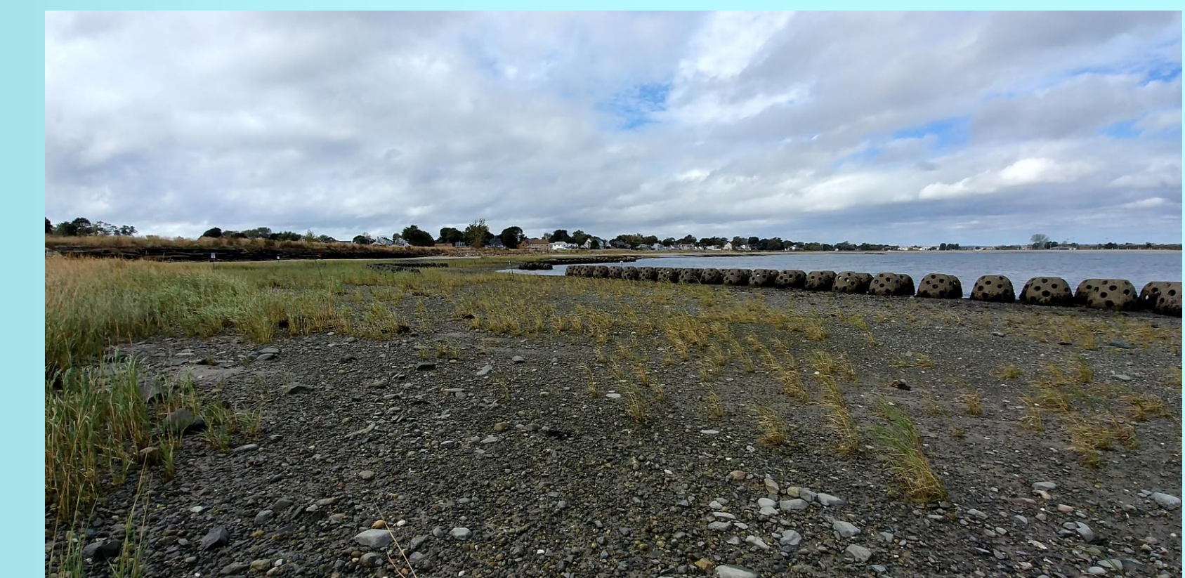
Figure 5. Restored marsh at Stratford Point showing exposed rock.
