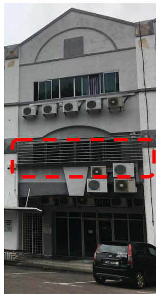
Fig. 1 - The installation of horizontal sun shading devices at the 1 st floor of Lot 105, Block A, City Campus Universiti Tun Hussein Onn Malaysia
