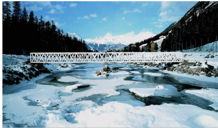
Figure 4. Pontresina Truss Footbridge, Switzerland [36,46].
