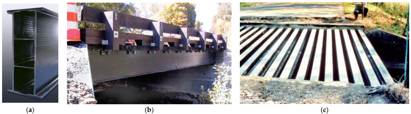
Figure 35. Pultruded FRP highway bridge girders [101]: (a) Strongwell EXTERN DWB; (b) Route 601 highway bridge in Sugar Grove, Virginia, USA using EXTERN DWB 900 \times 450 mm, built in 2001; (c) Tom's Creek Bridge, Blacksburg, Virginia, USA, built in 1997 and used EXTERN DWB 200 \times 150 mm.
