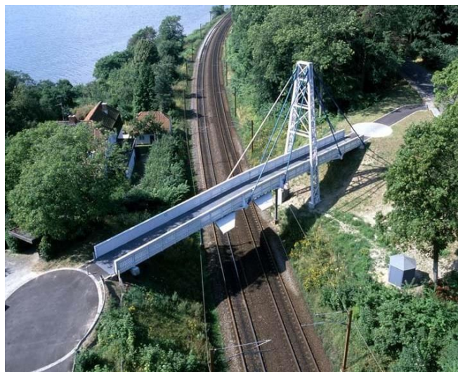
Figure 3. The 40 m Fiberline Composites bridge in Kolding, Denmark [46].
