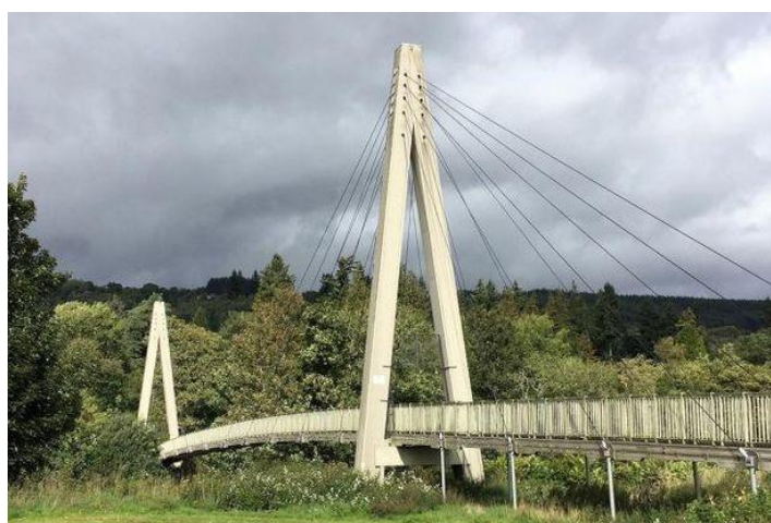
Figure 1. Aberfeldy cable-stayed pedestrian bridge, Scotland [42].
