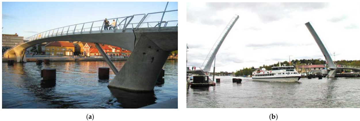
Figure 8. Fredrikstad Bascule Footbridge Norway, built in 2003 [55]: (a) Bridge in a closed state; (b) Bridge in an open state for navigation.
