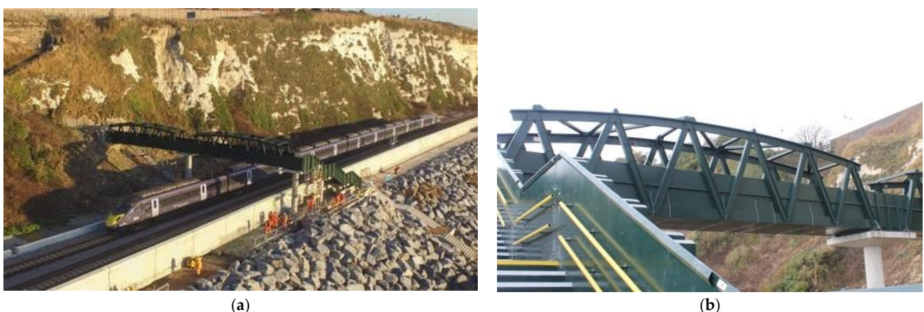
Figure 15. Dover Sea Wall Footbridge, Dover, Kent, UK, built in 2017 [64]: (a) Complete footbridge over a railway line; (b) Bridge span directly on top of rail tracks.
