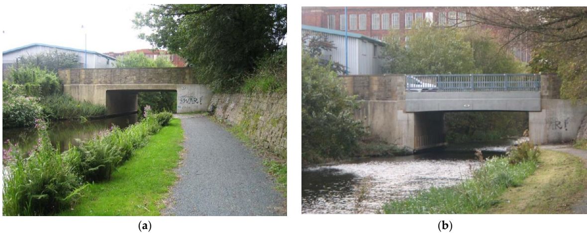
Figure 20. Moss Canal road bridge, Rochdale, UK, built in 2011 [72]: (a) Original bridge with in situ concrete portal frame; (b) New FRP bridge using double web pultruded FRP beams and FRP deck with multiaxial E-glass fibres.
