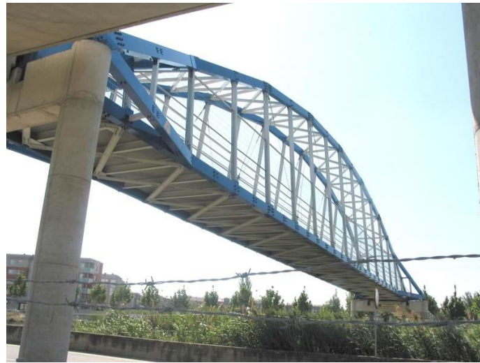
Figure 6. Lleida Footbridge, Spain, 2001 [50].
