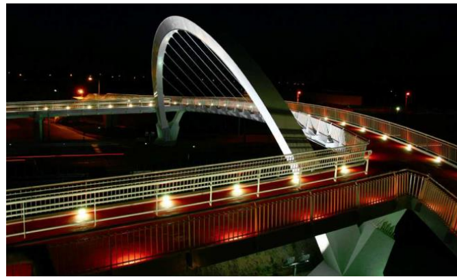
Figure 19. Gądkki Footbridge, Poland, built in 2008 [71].
