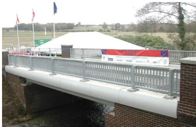
Figure 7. West Mill Bridge, Oxfordshire, UK, 2002 [52].
