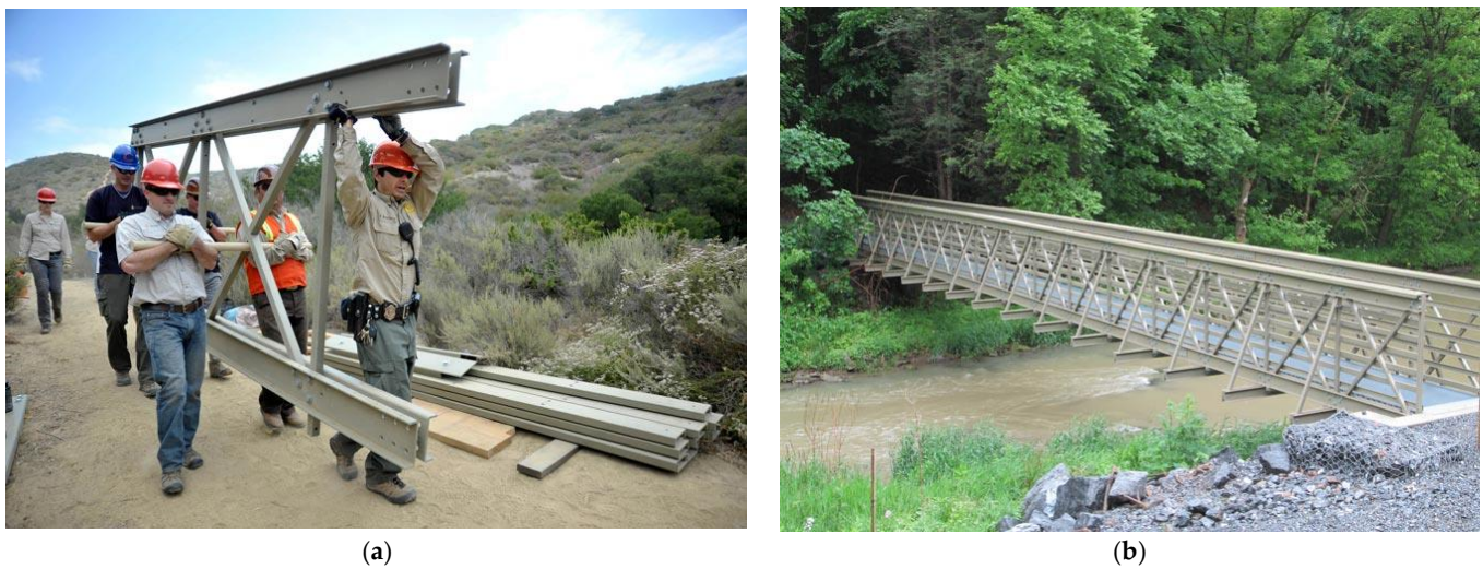
Figure 36. FRP light truss bridges [3]: (a) FRP truss ready to install; (b) Full FRP truss bridge.
