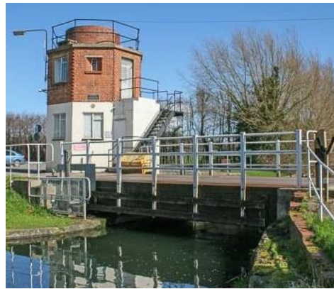
Figure 2. Bonds Mill Lift Bridge over the Thames–Severn canal in Gloucestershire, UK [40].
