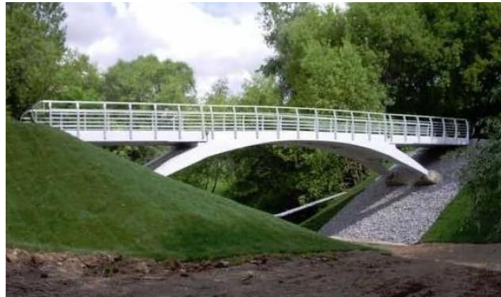
Figure 10. ApATeCh arched footbridge, Moscow, Russia, built in 2008 [39].
