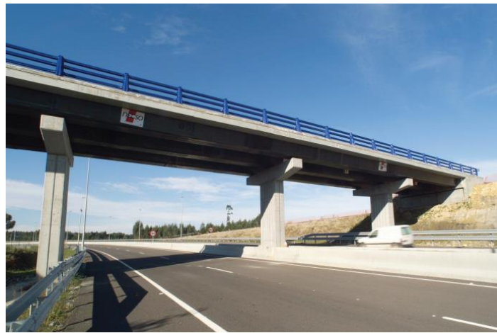
Figure 16. Asturias composite bridge CFRP girders and concrete deck, Spain, built in 2004 [66].
