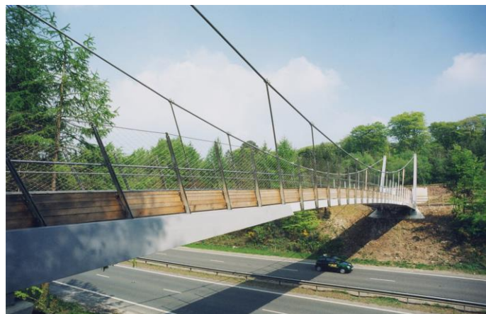
Figure 5. Halgover Footbridge, Bodmin, UK, 2001 [49].
