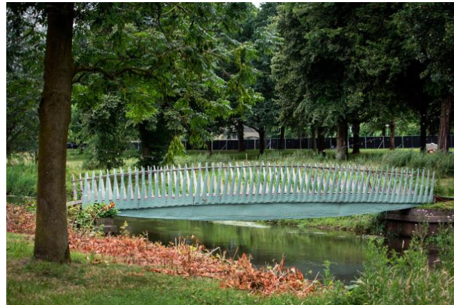
Figure 14. Eindhoven bio-composite footbridge over the river Dommel, Eindhoven, The Netherlands, built in 2016 [63].
