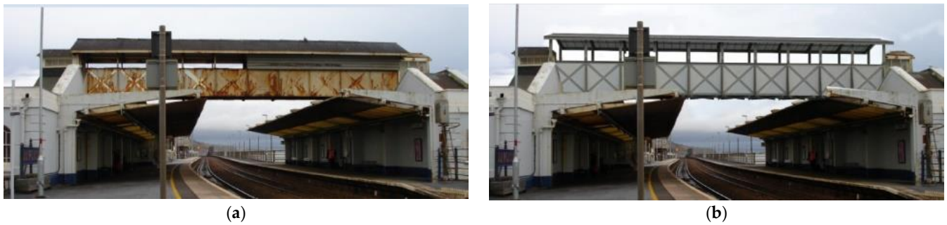
Figure 12. Dawlish Railway Footbridge, Exeter, South Devon, UK [1]: (a) Old rusty steel bridge using riveted built section and cross bracing, 1937; (b) New FRP bridge using pultruded FRP profiles, moulded parapet and stairway, 2012.
