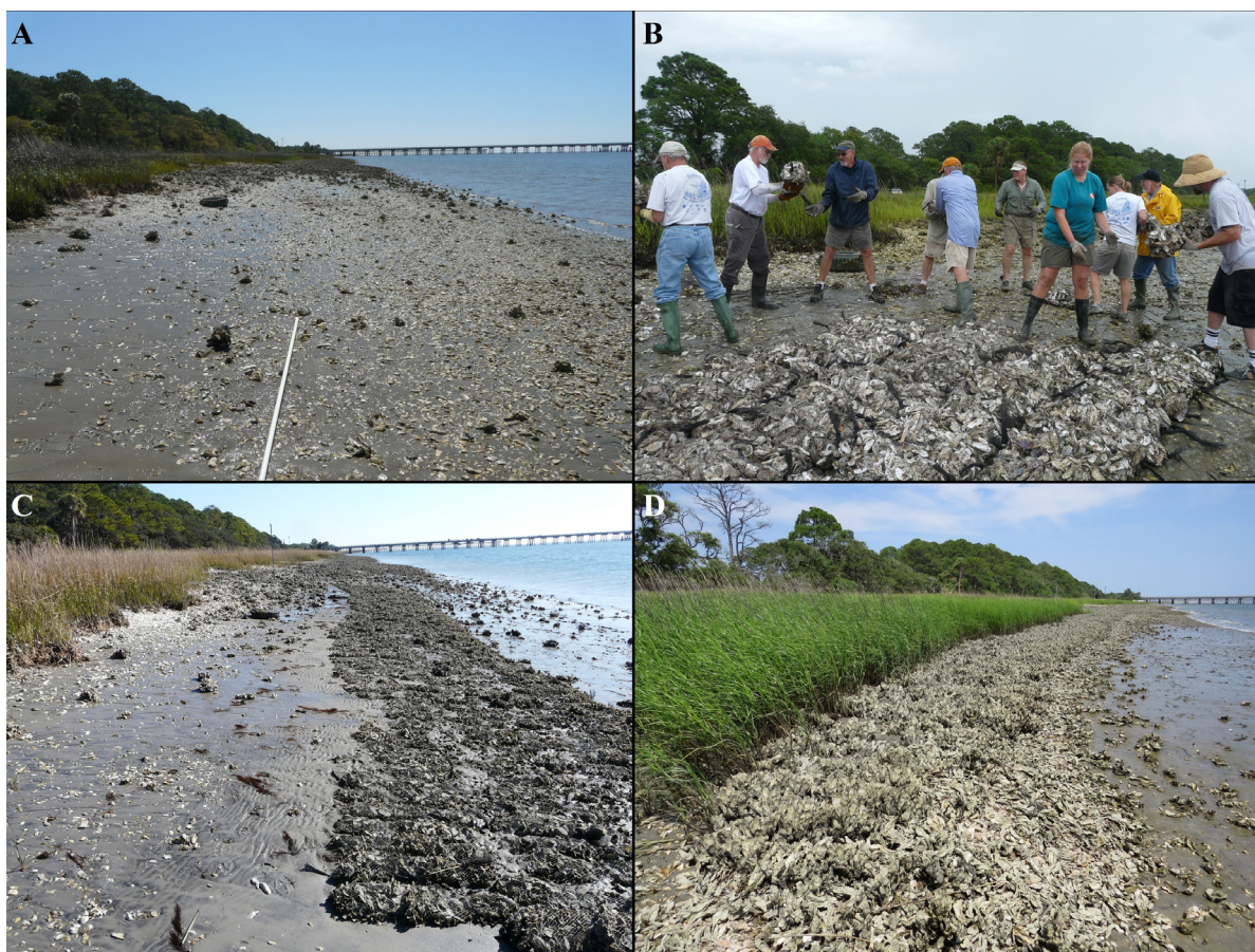
Figure 1. Time series of photographs from the SCDNR South Carolina Oyster Recycling and Enhancement (SCORE) Program site on Hunting Island, South Carolina (32.34467°N, 80.46765°W), illustrating the ability of intertidal bagged oyster shell reefs to facilitate salt marsh ( Spartina alterniflora ) habitat expansion. (A) April 21, 2009: Pre-installation condition of shoreline; note the lack of suitable substrate for oyster recruitment. (B) June 4, 2009: Creation of an intertidal bagged oyster shell reef through the addition of 400 shell bags (0.016 acres) by volunteers. (C) January 12, 2010: Approximately seven months post-installation. Sediment has begun to accumulate on the marsh side of the reef. Mean ( \pm SE) oyster recruitment at this time was measured as 4,693.3 \pm 749.1 oysters m^{-2} . (D) June 13, 2013: Approximately four years post-installation. The salt marsh has grown seaward, as much as 10 m, to the back of the reef, without any directed planting of S. alterniflora .
