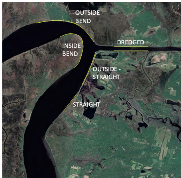
Figure 3. Illustration of categories of shoreline morphology used to investigate the effect of this site characteristic on reef performance metrics. Imagery was obtained from Google Earth, dated October 10, 2016, and includes sections of the Intracoastal Waterway and South Edisto River, South Carolina.
