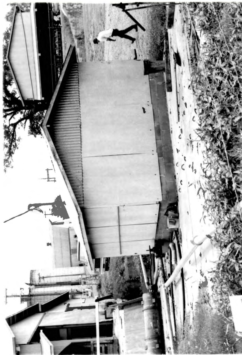
Figure 5. Manure Slurry Pumping Facility: Pump house located on manure tank and irrigation line (arrow) from pump house to plot.
